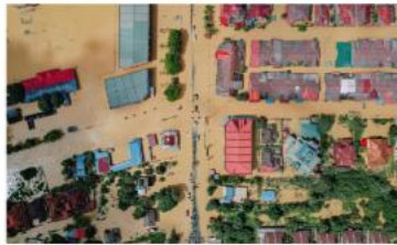
assessing flood damage
